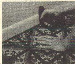
Tredway installs with staples.
